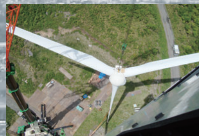
Wind turbine installation
