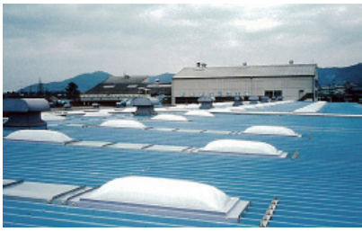
Skylights at Toyotsu-new Pack
