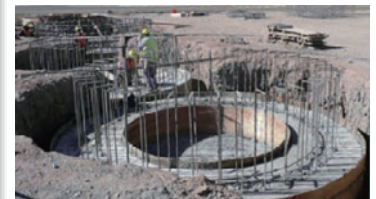
Lime plant under construction
