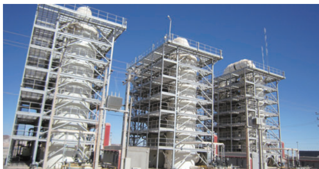
Iodine is extracted and condensed using a blowout tower located in the middle of a desert.
