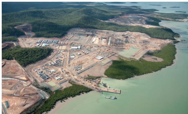
LNG conversion plant underway near the port of Gladstone
