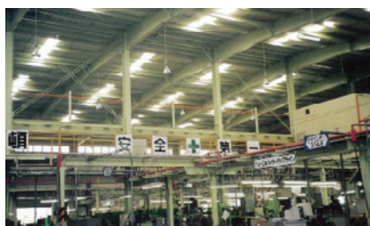
Skylights at Toyotsu-new Pack (upper: external view; lower: inside view)
