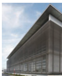
Louvers for protection from sunlight (Toyota Branch)
