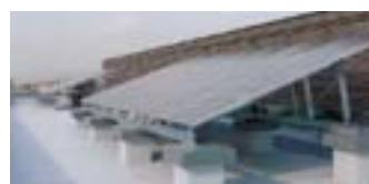
Installation of solar power generation system
