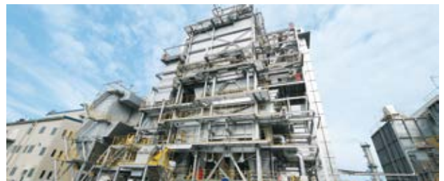
Ehime Prefecture's first biomass power plant
