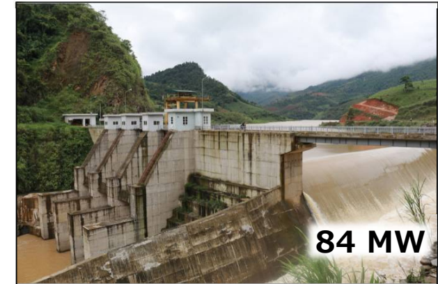
Ngoi Phat Hydropower Plant (Vietnam)
