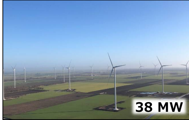
Windpark Mondriaan (Netherlands)
