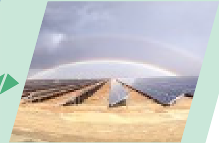
Establishment of AEOLUS renewable energy project in Africa
