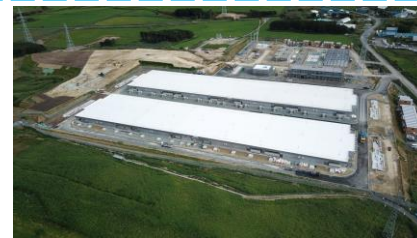
Northern Hokkaido storage batteries business
