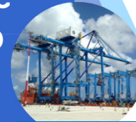
Port Cargo Handling Cranes
