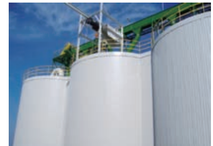
This New Silo was Built at Toyo Grain Terminal Co., Ltd.
