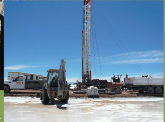
▶ Brine production well excavation
