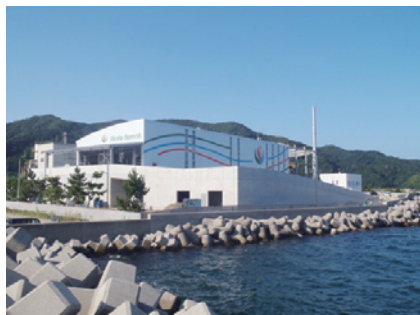
Sewage sludge carbonization plant of Waste Biomass Co., Ltd. commenced full-scale operations from April 2013.
