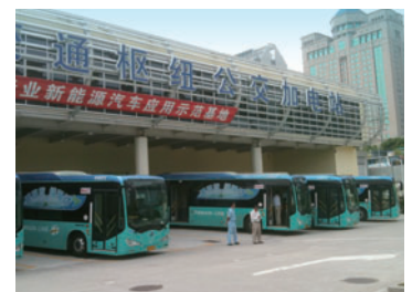
EV bus charging station operated by Chinese partner Potevio New Energy Co., Ltd.
