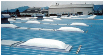
Skylights at Toyotsu-new Pack
