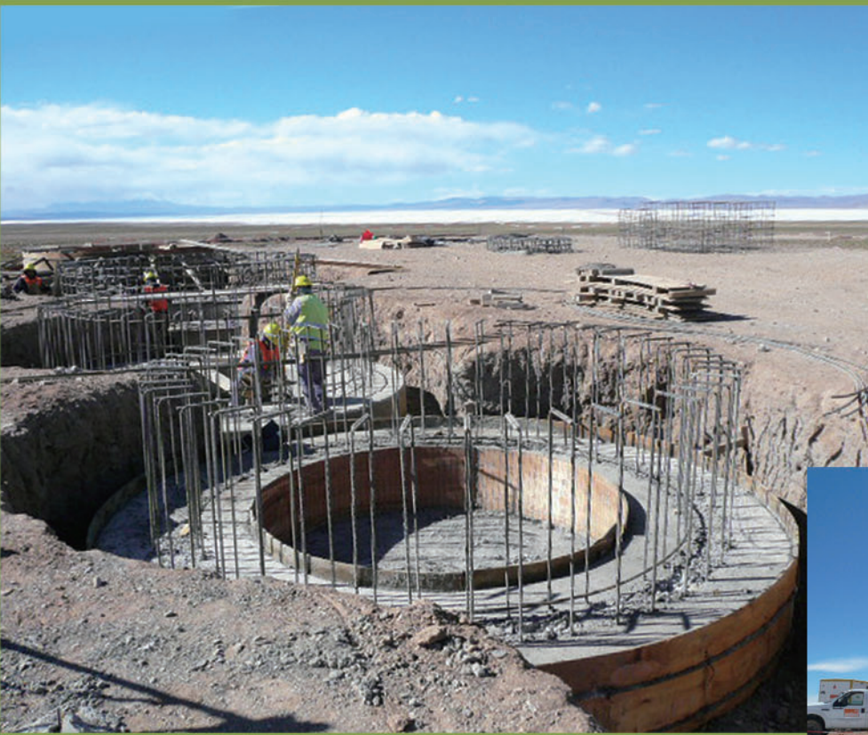
▲ Lime plant tanks under construction
