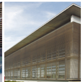
Installation of louvers
