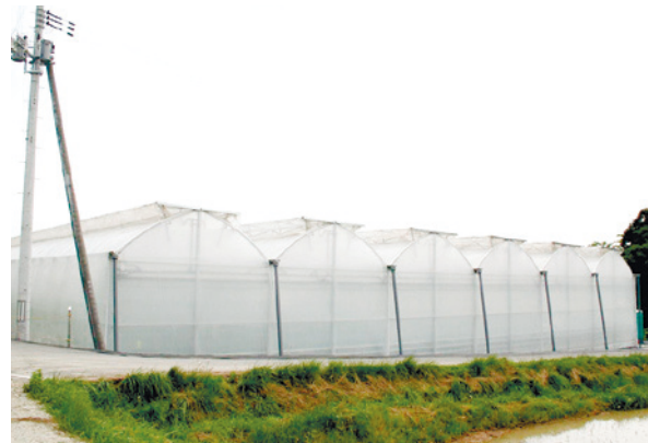
Large steel-frame greenhouse facility (commonly referred to as the “Air House”)
