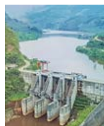
Ngoi Phat Hydropower Plant (Vietnam)
