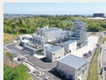
Toyotsu Lithium's Naraha Plant under construction
