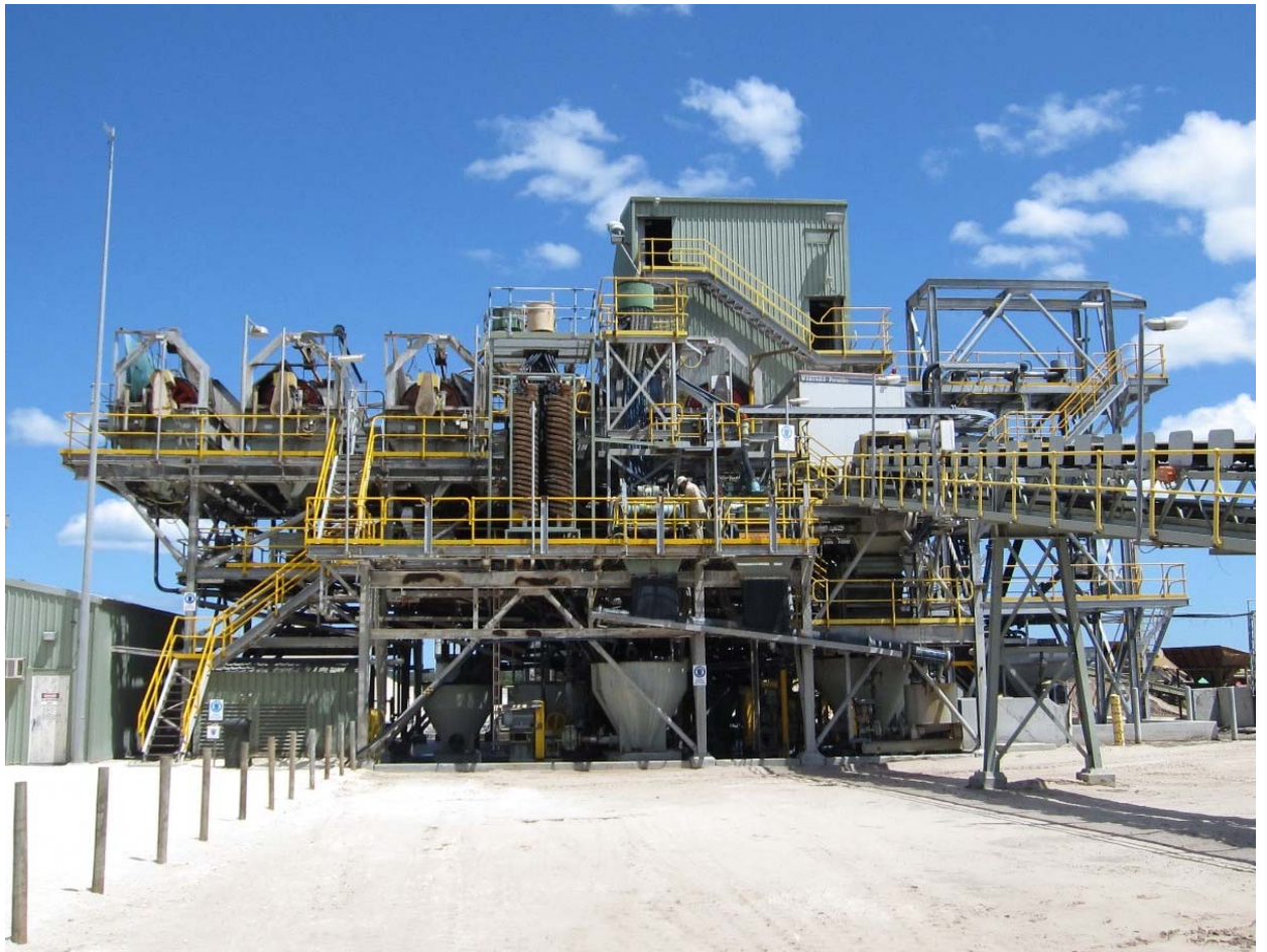
(Silica sand refinery)
